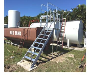
Carmen McKinney was pleased with the work of the above project at the Winkler Helistop. It is a set of stairs that connect the Mix Tank with the Jet Fuel Tank that Chuck Herzog and Tom Peters designed and fabricated in-house. The job turned out wonderfully. Kudos guys.
