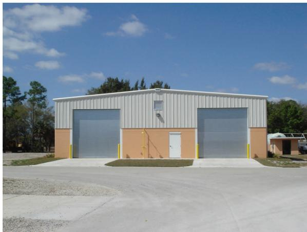
The mix/load building was completed in December. Pesticide mix-load facilities are designed to eliminate environmental contamination while sprayers are being filled with water and product and also designed for containment and recovery of spilled pesticides and herbicides.
